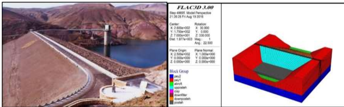
Fig. 2. General view of Sattarkhan Dam and its3D modeling
