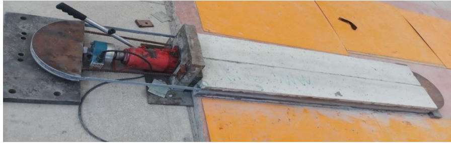
Fig. 2. Prestressing of NSM CFRP
