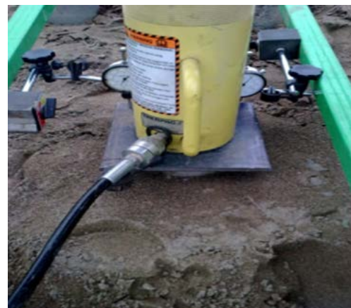
Fig. 3. Pile displacement measurement gauges
