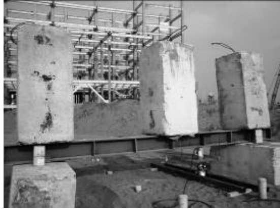
Fig 1. Placement of blocks on the beam
