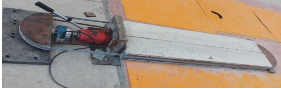
Fig. 2. Prestressing of NSM CFRP
