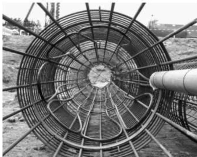
**Fig. 1.** Absorber pipes fitted to the reinforcement cage of a large-diameter bored energy pile (Brandl, 2006)
